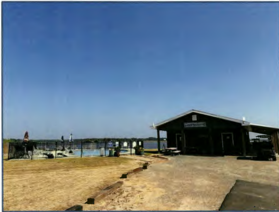
General ground view of subject property (RV clubhouse & office)
