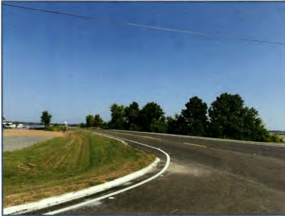
Street view along MS Highway 43 facing northward
