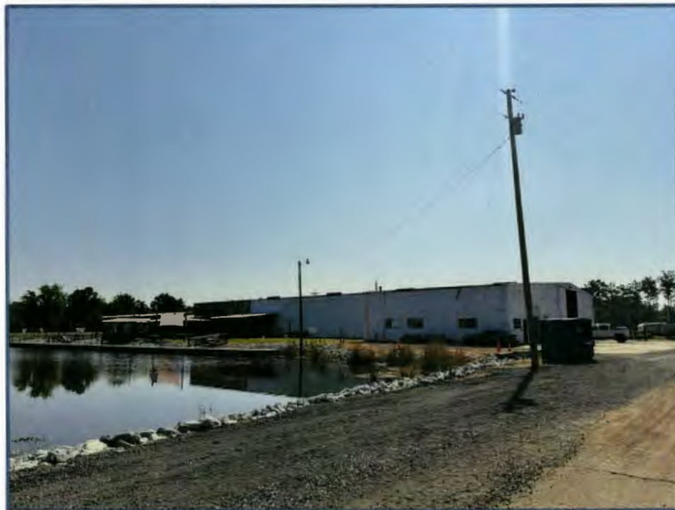
General ground view of subject property (industrial/retail building)
