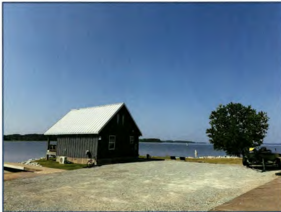
General ground view of subject property and Barnett Reservoir frontage
